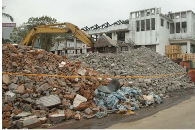
All that remains of the Sasakawa Memorial Hall is rubble. In the background is the historic theater building, which is also being demolished.
