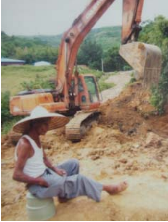
Lu De Chang tries to block the destruction of Lo Sheng. Photo Courtesy Lu De Chang
